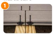
Place 4 clips centered on joist on both sides of the boards.
