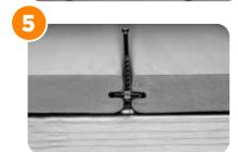
Slide the clips (screws and gussets) down the groove, positioning one over each joist on both sides of the board.
